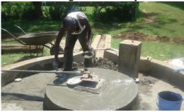
Sealing the well after pump was installed
