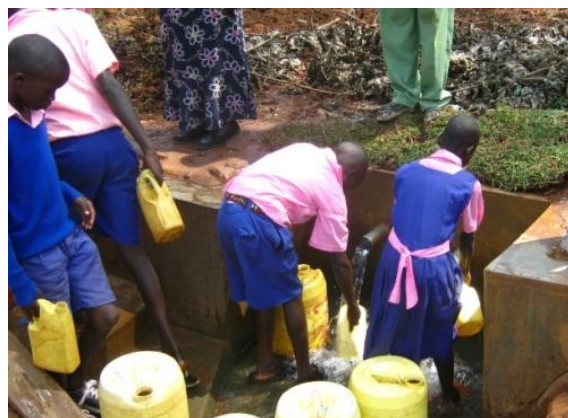
Sample photo of a protected spring with outlet pipe
