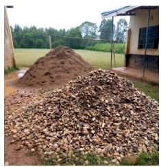
Sand and ballast for the water tank base
